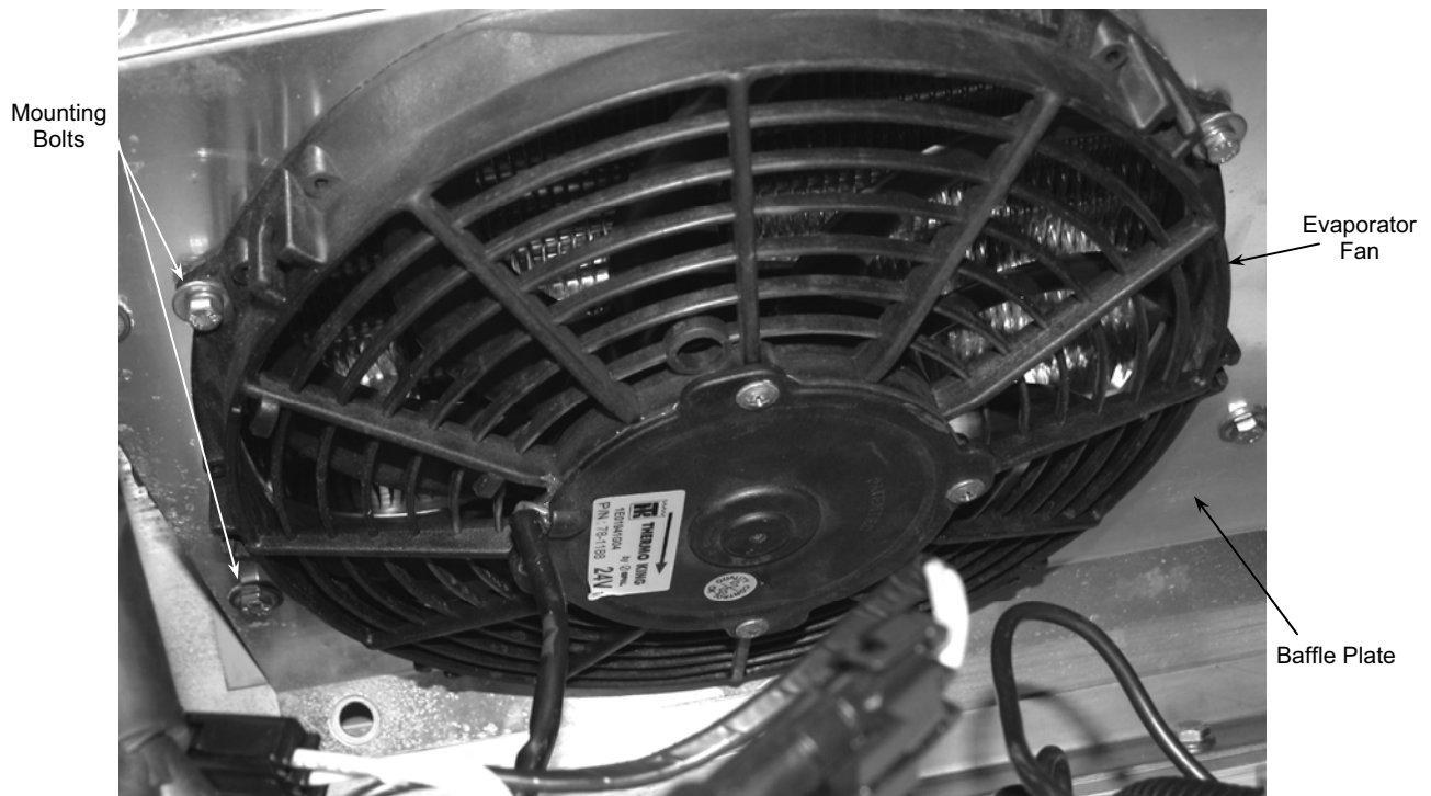
Figure 1. Evaporator Fan.
