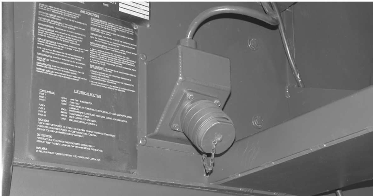
Figure 4. Cannon Plug (RU Power Supply).
