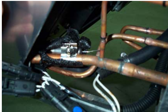
Figure 1. Sensing Bulb.
