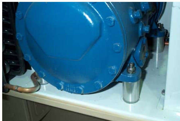
Figure 1. Oil Drain Plug.
